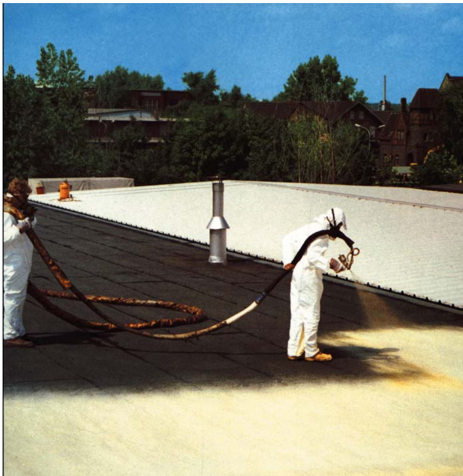
Fig. 37: Thermal insulation and sealing in one operation
