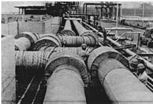
Figure 5.38 LPG Pipelines by Frothing-in-Place, [5.44].
