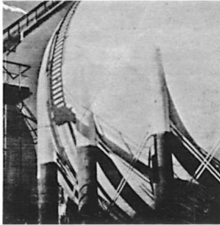
Figure 4.12 Spherical LPG Tank Insulated by Frothing-in-Place [4.54].
