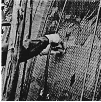
Figure 4.13(b) Frothing-in-Place Operation onto Tank Surface [4.54].
